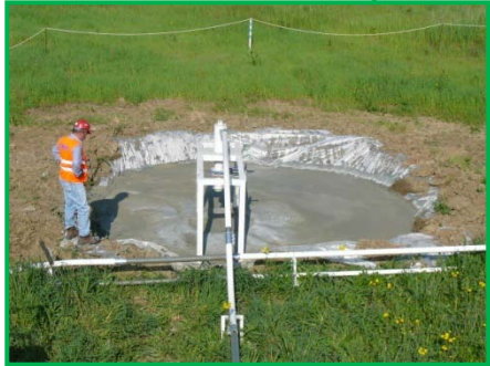
Trevi SpA - Pilot Plant
