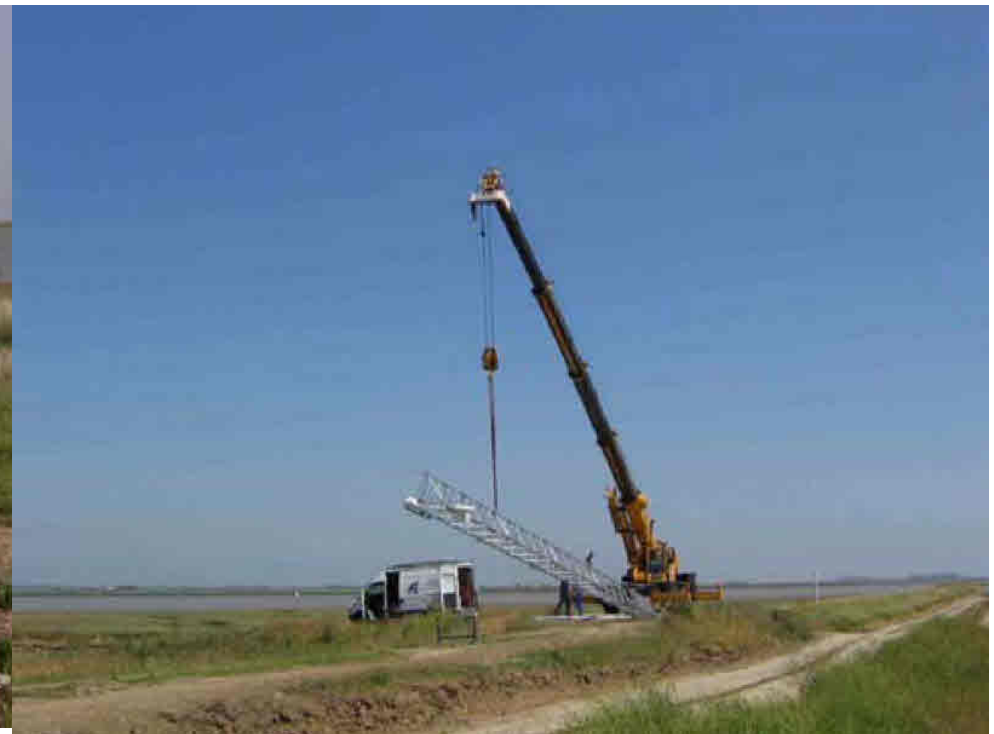
Web camera tower being erected
