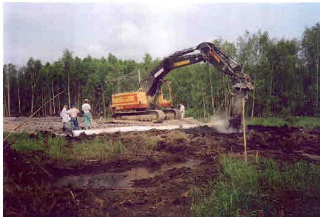
Mass stabilisation in Veittostensuo 1993
