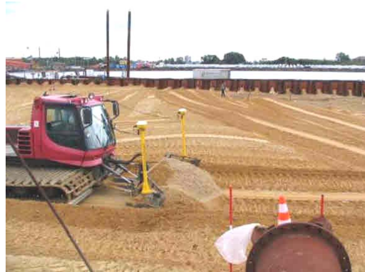
placing of (dry) Sand by PistenBully
