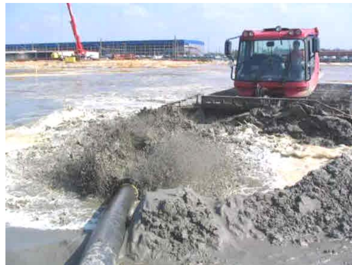
placing of sand flushing method
