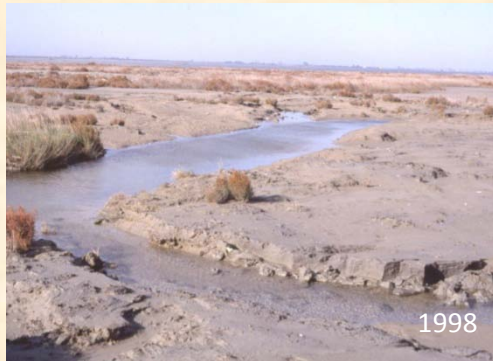
Excavation of a creek and pond in salt marsh Chioggia B1
