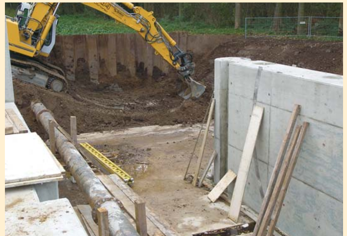
The weir, under construction
