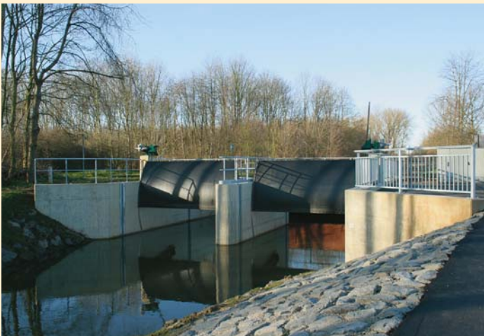
The weir, completed
