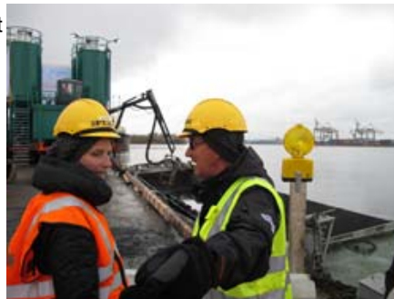
Port of Gävle during stabilisation/solidification of contaminated sediments
