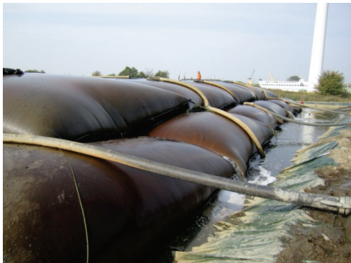
Fig. 1: Installed tubes in a pyramidal pattern.
