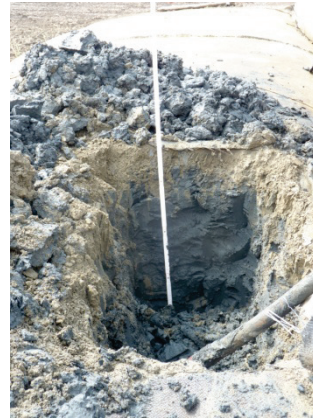
Fig. 2: Trial pit in the lower (first) tube layer.
