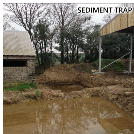
Sediment trap and infiltration drainage pond created to prevent sediment from agricultural land entering the local river
