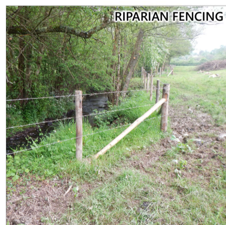
Riparian fencing erected to prevent livestock from entering the river and to encourage vegetation recovery
