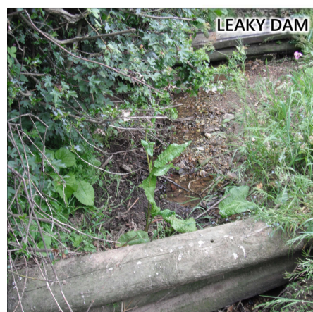
A series of leaky dams constructed to slow water flow and encourage sediment deposition
