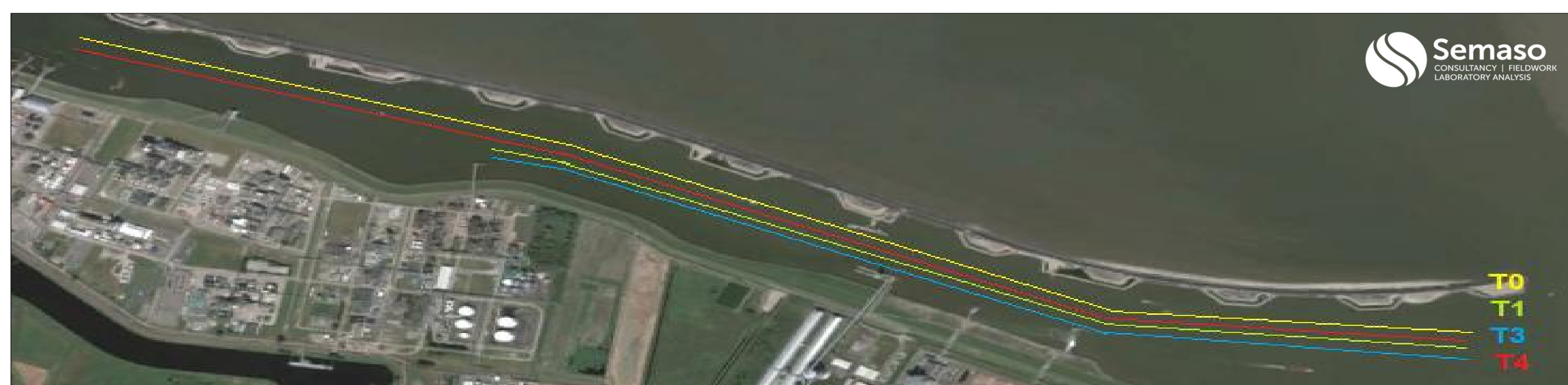
Fig.1 Aerial view of the entrance channel of the port of Delfzijl
