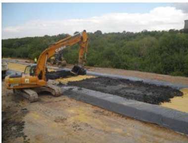
Fig. 1: Subgrade road layer manufacture
