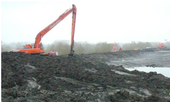
Fig. 1: Sediment used as a resource for further reallocation in fluvial civil works.
