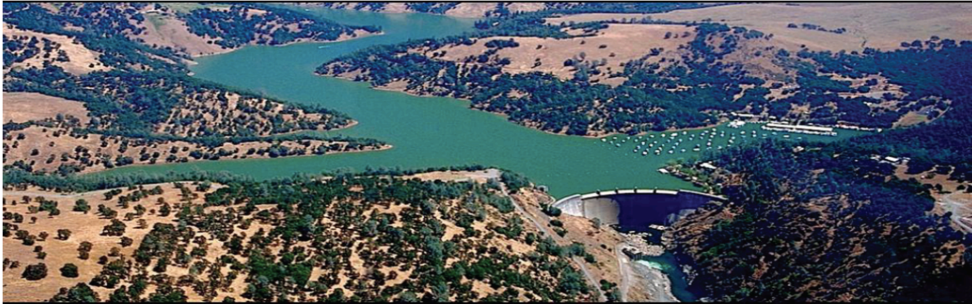
The reservoir above Englebright Dam on the Yuba River—a third filled up with sediment.
