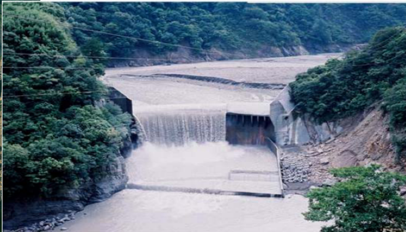
Sept 2004 - dam full of sediment
