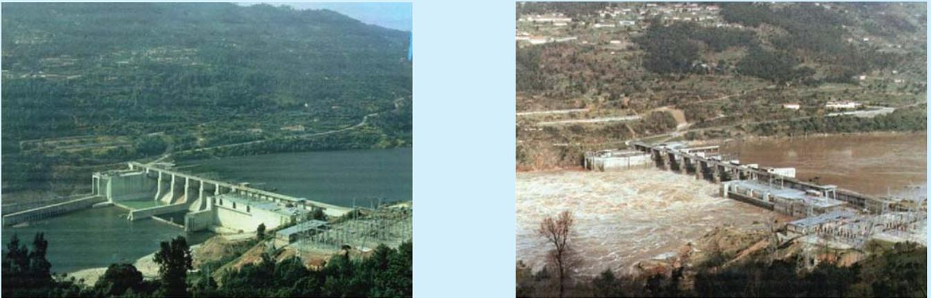
Figure 5 Carrapatelo dam during average hydrological conditions (left) and during the flood event of 1978 (courtesy of F. Veloso Gomes)
