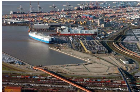
Fig. 1: a new handling area for automobile export in Bremerhaven, Germany.
