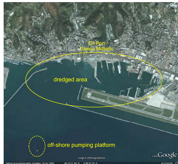
Fig. 1: Area of the Oil Port of Genoa Multedo: the yellow ellipse represents the dredged area and the broken yellow ellipse the position of the damaged off-shore oil platform.
