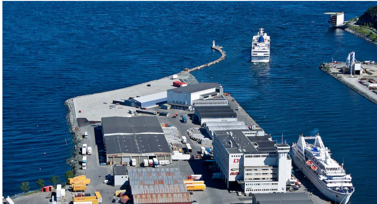
CDF after completion in Trondheim harbour. Photo Åge Hojem/Trondheim harbour
