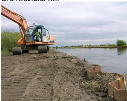
Fig. 1: Sediment re-used as structural fill.
