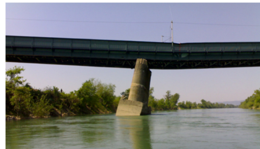
The railway bridge Jakuševac in Mičevac on the Sava River that collapsed on March 30, 2009
