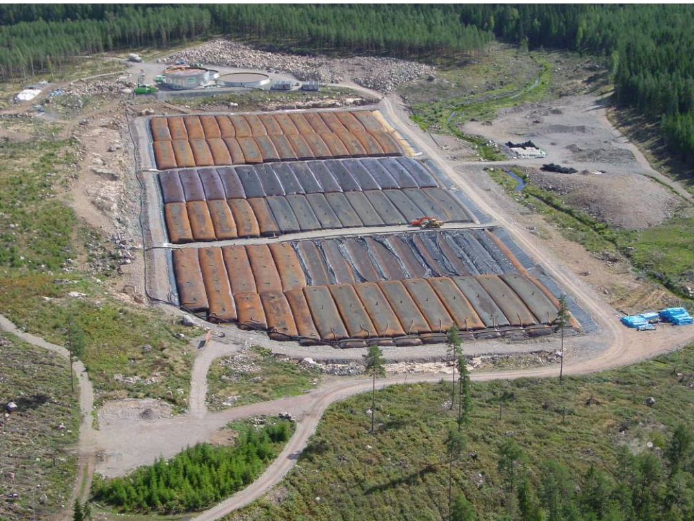
Aerial view on the landfill site with the filled geotubes.
