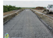
Impermeabilisation using a layer of stone-based asphalt after compaction
