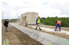
Addition of lime using a spreading truck
