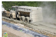
Addition of binder using a spreading truck
