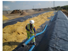
Geomembrane, recovery drains and neutral sand
