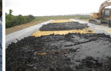
Spreading sediments
