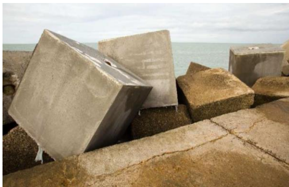
Fig. 1: Sediment used in concrete for coastal defence blocks. SEDIMATERIAUX, port of Dunkirk.
