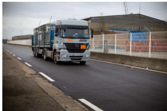
Fig. 2: Sediment used in harbour road base. Ibid.
