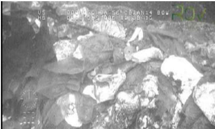
Exposed waste due to damaged cap at Kollevågen (NGI, 2014)
