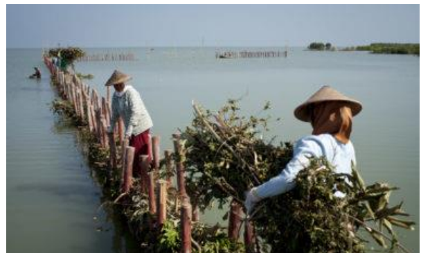
Fig. 1: Permeable dams at the Demak site, Indonesia .
