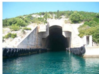
Figure 1: Location of underground military harbor “Papratna”, Island of Dugi otok. and photo of harbor entrance.
