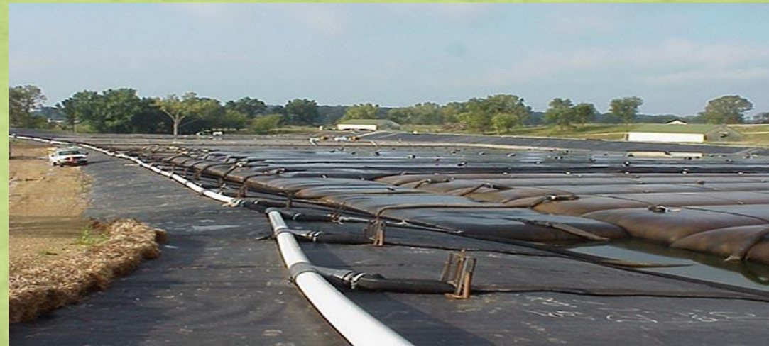
Boskalis – Membrane Dewatering Lower Passaic River, New Jersey
