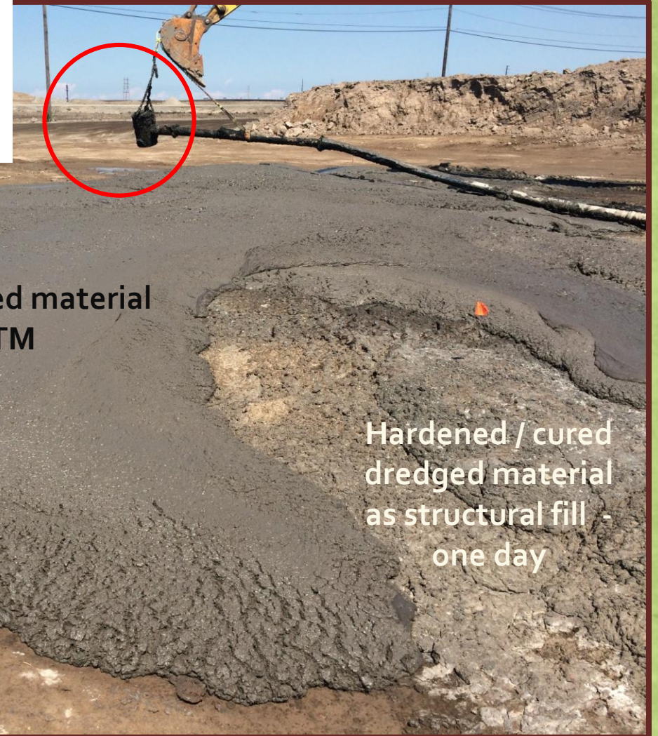
Pneumatic Tube Mixing for Contaminated Soft Sediments
