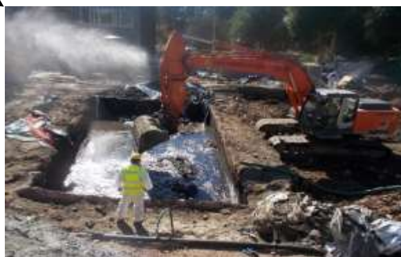
Former gasification plant
