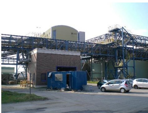
Fig. 1: CUTEC pilot plant at the METHA II plant
