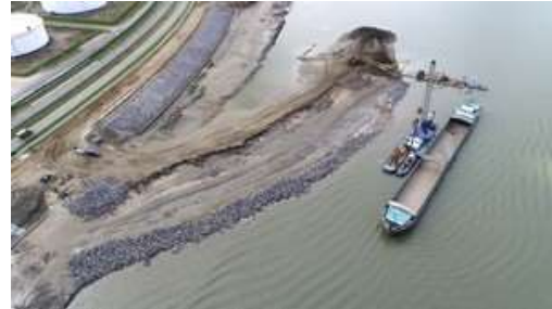
Fig. 2: Groyne during construction phase.
