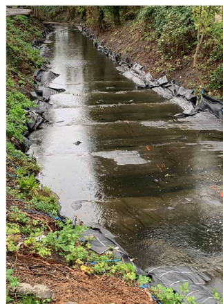
Fig. 1: Placement of reactive mat in the Lieve
