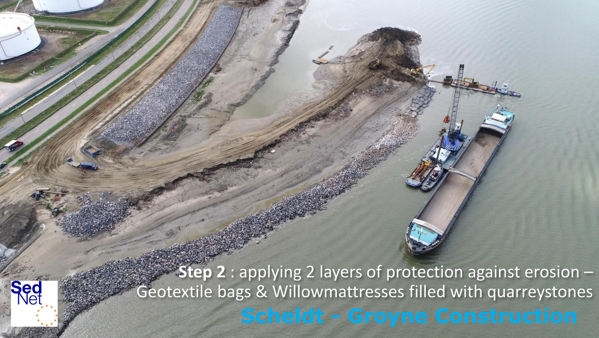
Step 2 : applying 2 layers of protection against erosion –
