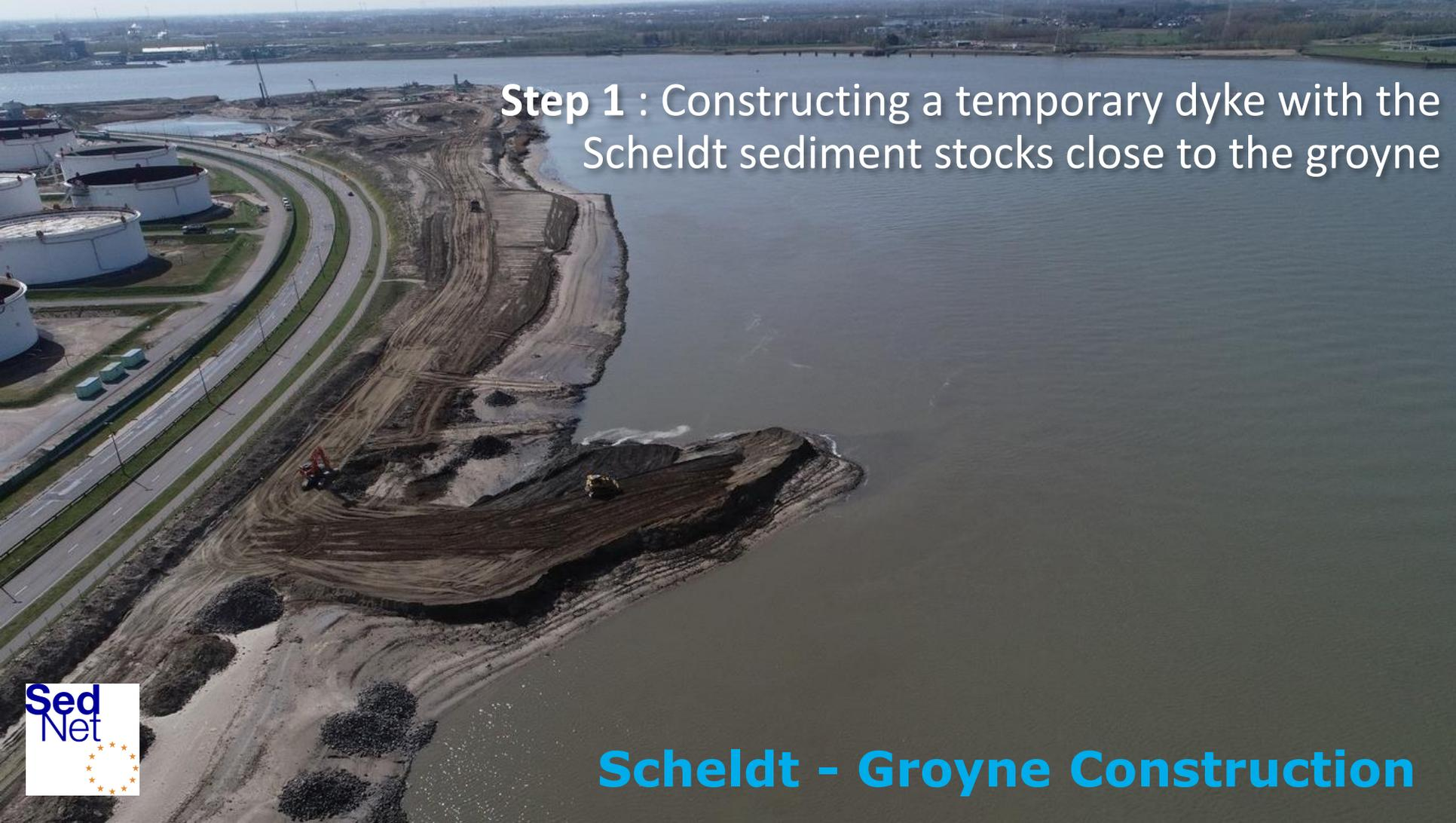
**Step 1** : Constructing a temporary dyke with the Scheldt sediment stocks close to the groyne
