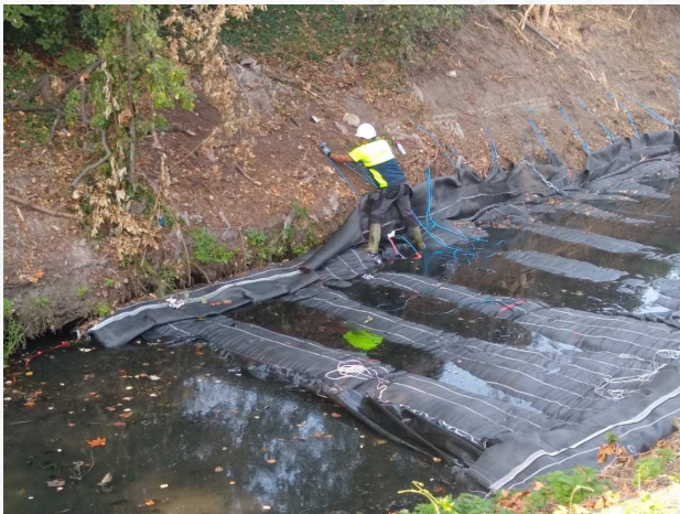
4. Anchoring to the bank
