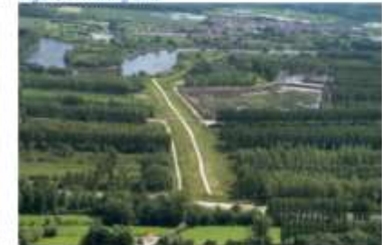
Figure 4. Finished Compartment dyke
