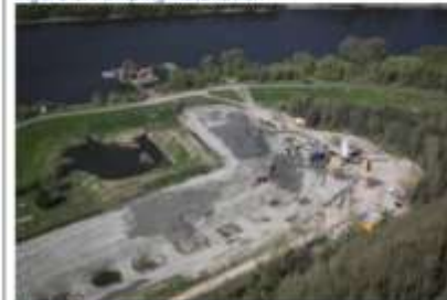
Figure 3. Site view during works
