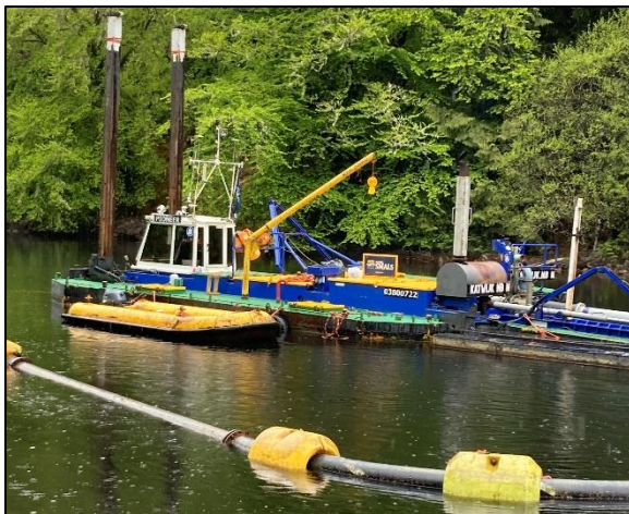
Fig.1: Suction dredging on the Caledonian Canal.
