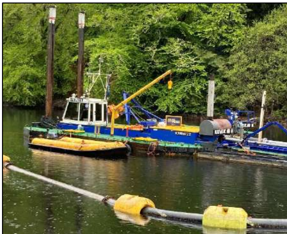
Fig.1: Suction dredging on the Caledonian Canal.
