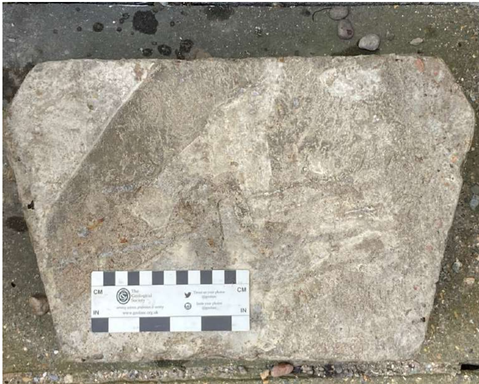
Concrete block for retaining wall – flood control
