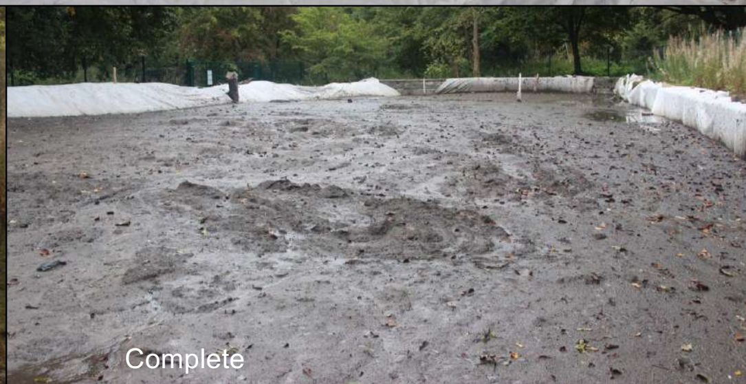
Basin lined with geofabric and wells installed
