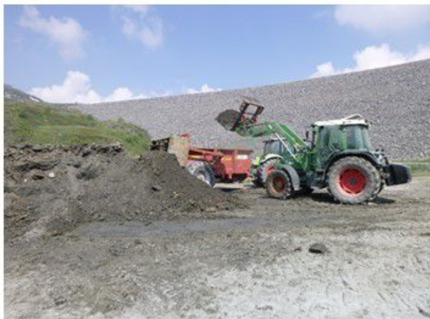
Spreading of the sediment/manure/compost mixture with 2 tractors, 1 loader and 1 manure spreader
