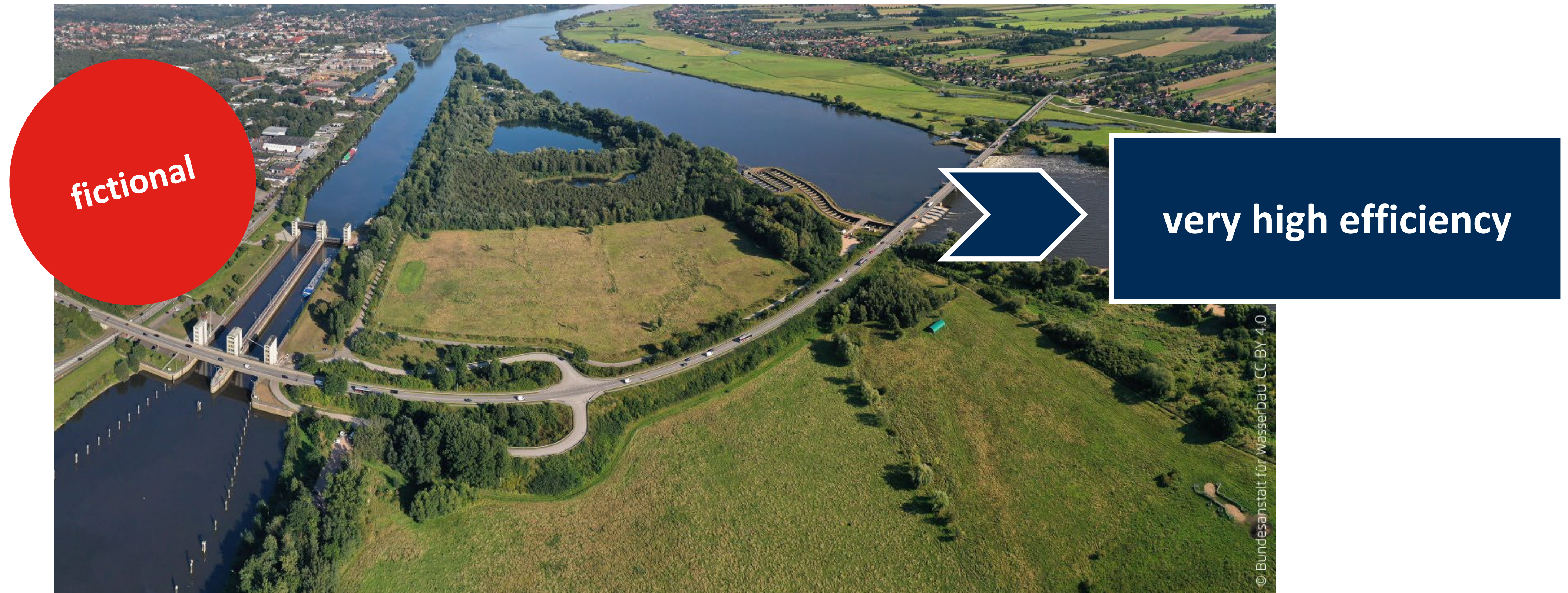
A weir with sedimentation basin serves as a fictitious measure for the socio-economic study. The structure could be similar to the weir and its sluices in Geesthacht, here aerial photo.
