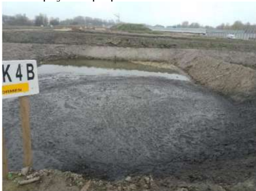
Fig. 1: One of the dewatering ponds after having been filled with dredged sediment.
