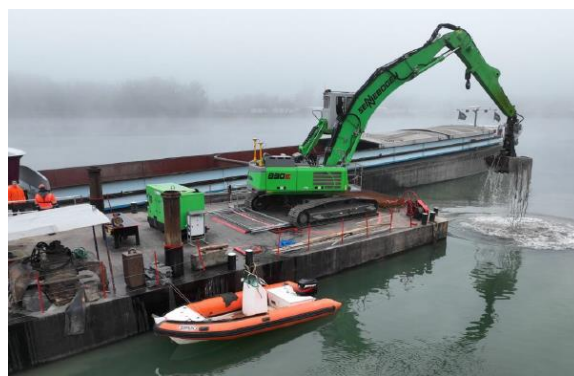
Fig. 1: Dredging sediments for reuse.
