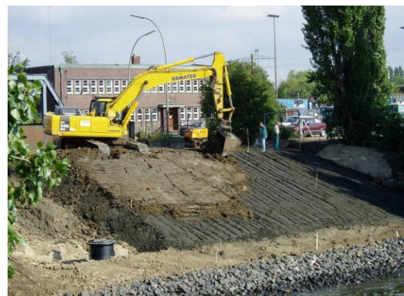
Fig. 1: Sediments beneficial use for dike construction, Germany.
