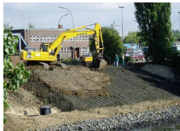
Fig. 1: Sediments beneficial use for dike construction, Germany.
