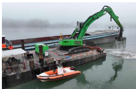
Fig. 1: Dredging sediments for reuse.
