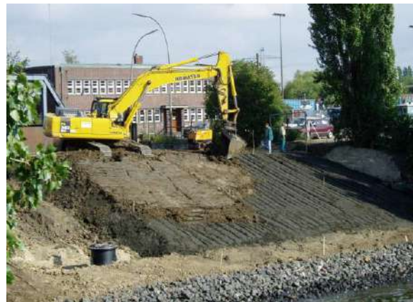
Fig. 1: Sediments beneficial use for dike construction, Germany.
