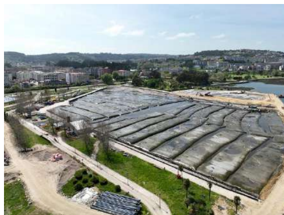
Fig. 1: Areal view of the confined dredging facility in Culleredo.
