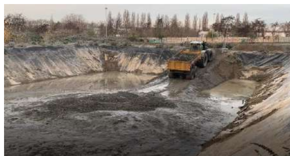
Fig. 2: Drying sediments is essential for recovery.
