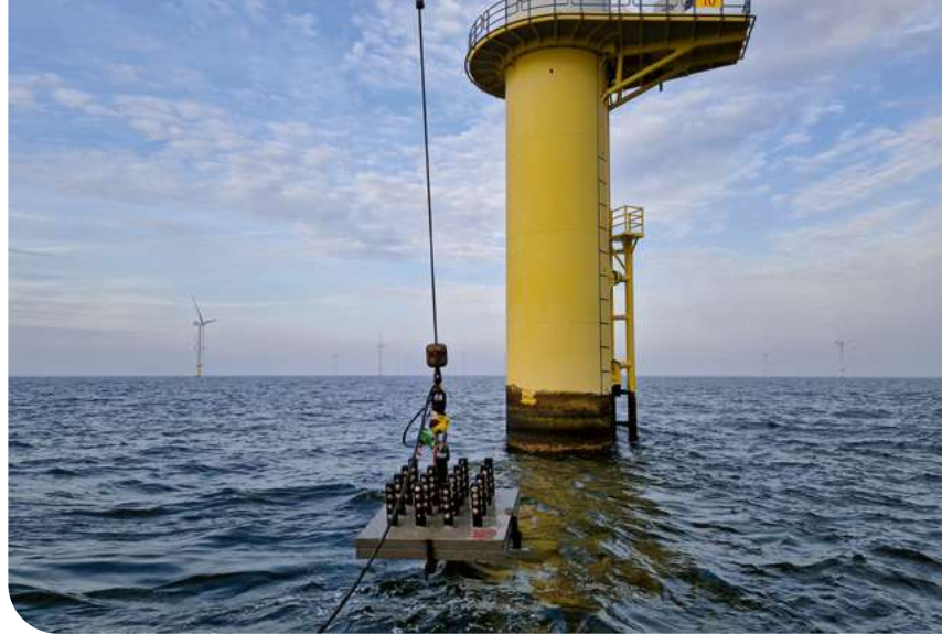
Oyster table installation at Luchterduinen offshore wind farm in the North Sea.
